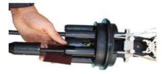
7: Using abrasive strip to rough the surface of the cable sheath and ports slightly.
